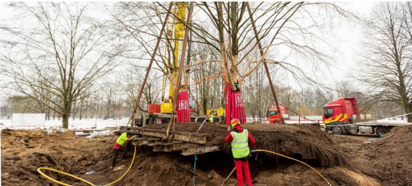
Figure 4 (Jēkabs Ozols, "Labie koki" Ltd., Latvia 2020). Large-size tree transplanting with manual root ball preparation and using heavy machinery.
