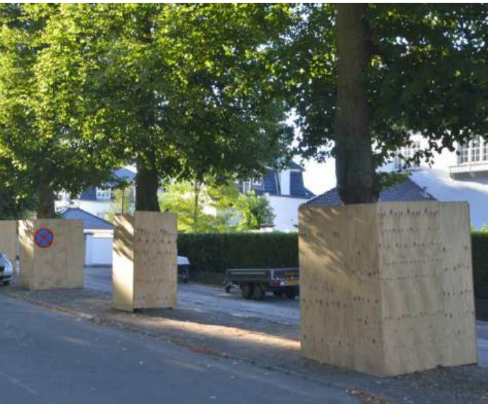
Figure 3 (C.C.N. Nielsen). Stem protection of trees surrounded by a permanent hard surface next to a construction site.
