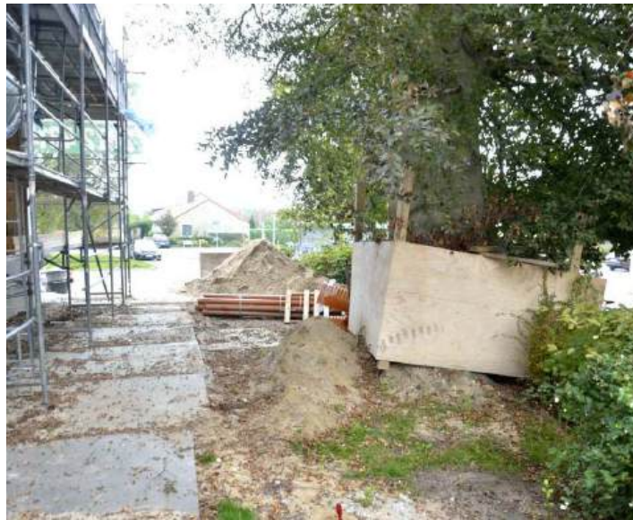
Figure 4 (C.C.N. Nielsen). The protection box has been pushed around and lifted in order to place remnant soil inside of it.
